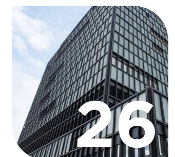
Multitec and National Projects Service Center
